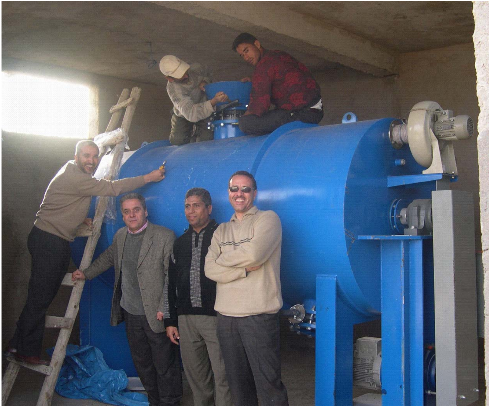
Assembling the Top part of the Bioreactor
