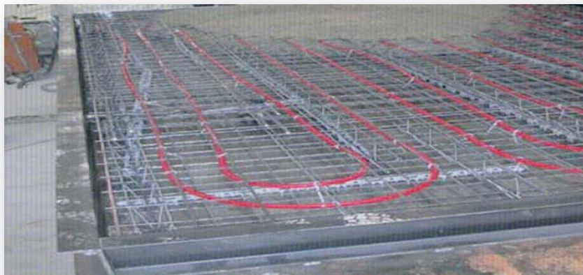
Picture 20.: Heat water pipes (Lazaretos.,2009)
