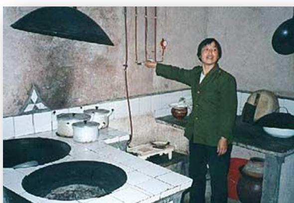
Picture 72.: Household biogas use for kitchen appliances
