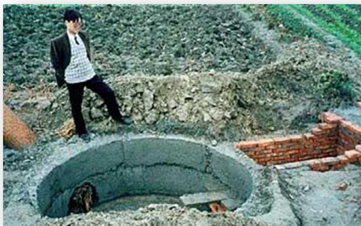
Picture 73.: Household (AD) under construction
