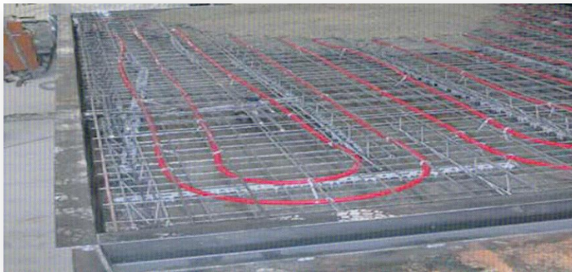
Picture.9: Heat water pipes (Lazaretos.,2009)
