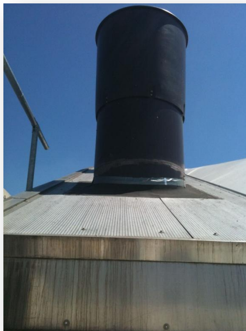
Picture.13: Air removal chimney
