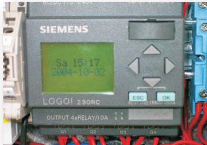
Picture.12: Programmable logical control system
